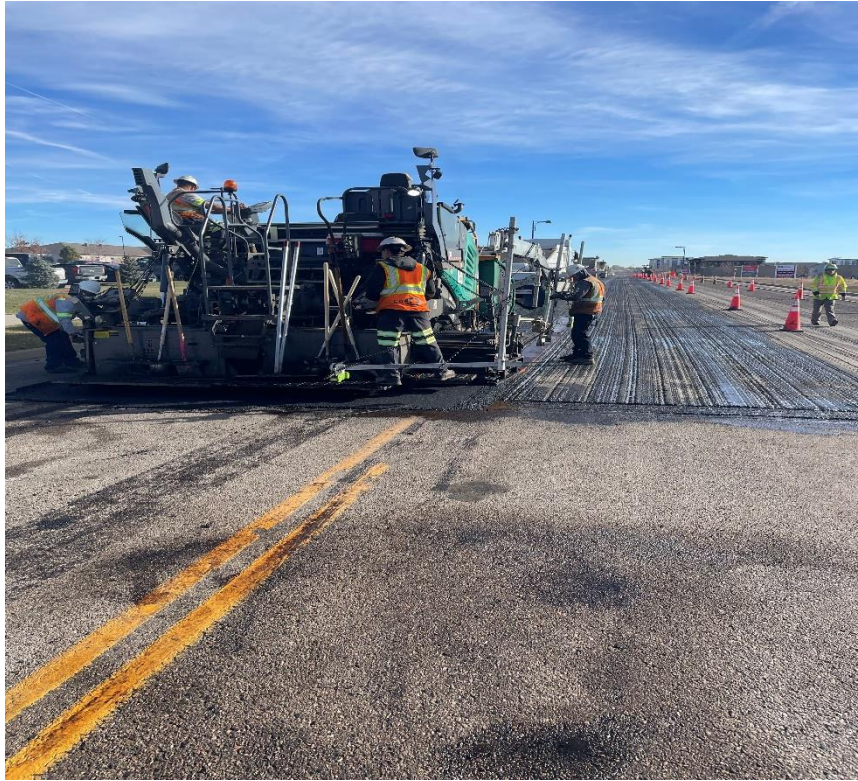
Roanald Reagan Blvd being paved.
