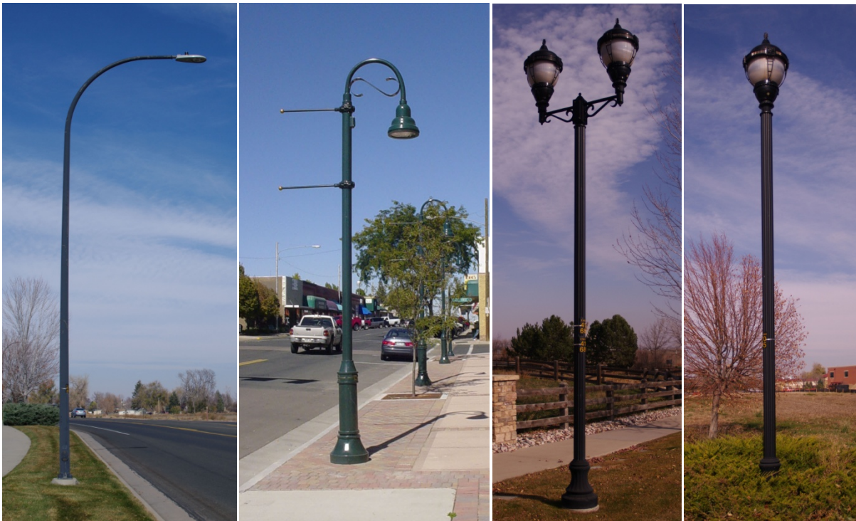
Examples of existing site & street lighting nearby.
